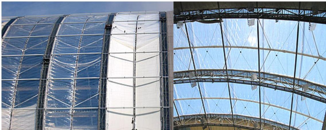
ETFE is the fluoropolymer-material ethylene tetrafluoroethylene which is used in structural membrane constructions in thicknesses from 0.05 to 0.25 mm.
